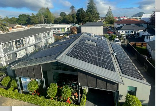
After monitoring the main grid and the facility for about three months, Guild & Spence determined a 29.5 kW PV system with 40kWh of battery storage was needed to satisfy these requirements. The system would provide up to 90 percent of the facility's power needs in the summer and 90 percent of their essential power needs in the winter, with enough capacity to still enable the daily benefit of the overall system.
