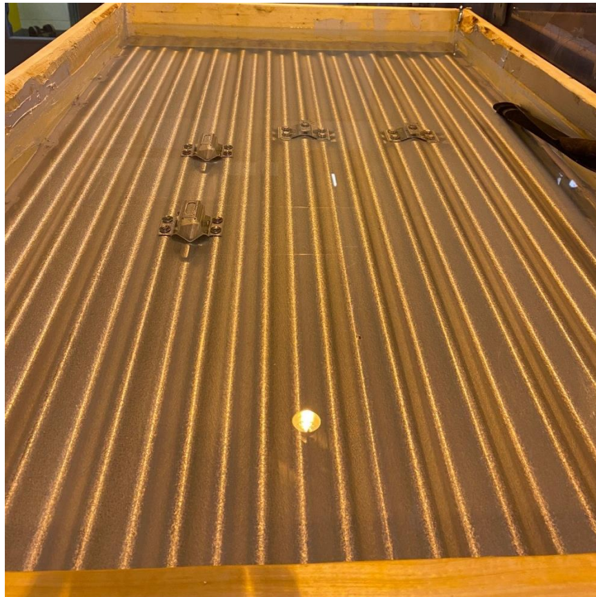
Photo No. 2 System #2
